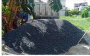
Provision of Agregates Construction Materials of Barangay San Vicente
